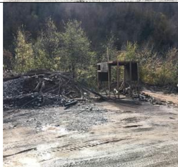
Spoil, timber, metal and concrete debris KM 44+800; 44+000; 44+200, 44+160; 42+480, 42+200. No hard barriers, no warning signs, improper housekeeping.
