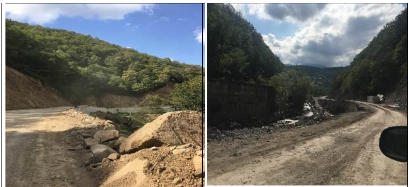
KM 13-14; KM 20 Deep cuts without hard barriers and warning signs
