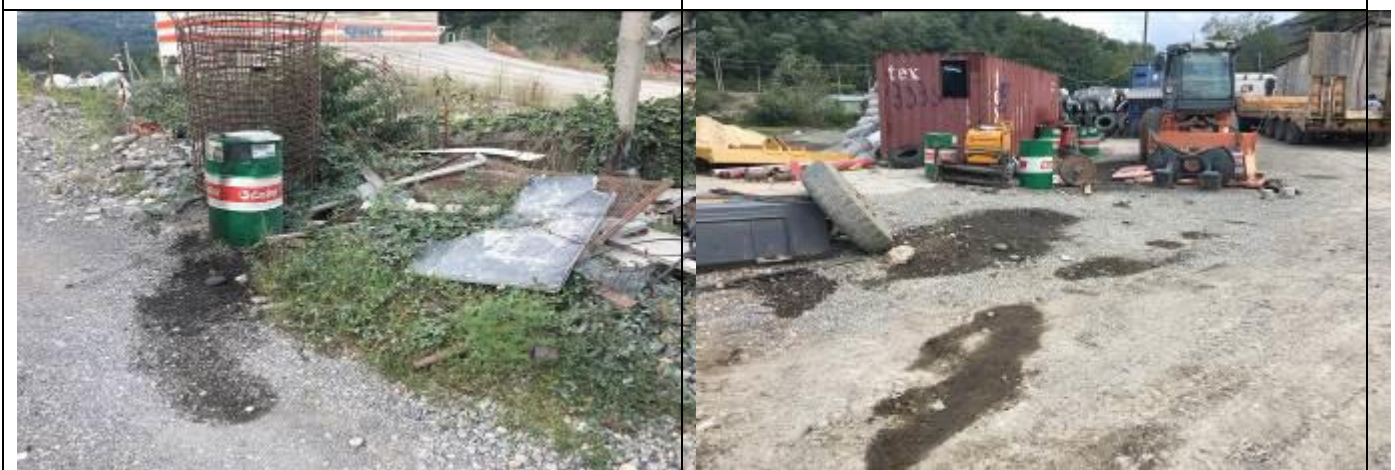
Unacceptable housekeeping and multiple oil spills, oil drums kept outdoor (Sagandzile Crusher area, Kharagauli camp)
