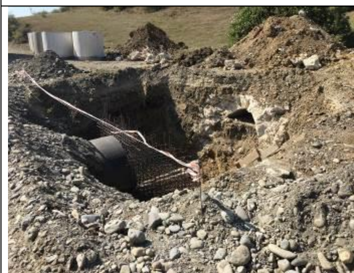
Spoil disposal area and concrete debris KM 48+600; 48+046; 47+800. No hard barriers, no warning signs, improper housekeeping
