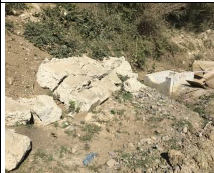
Spoil, timber, metal and concrete debris KM 44+800; 44+000; 44+200, 44+160; 42+480, 42+200. No hard barriers, no warning signs, improper housekeeping.
