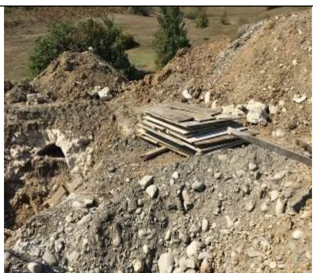
Spoil disposal area and concrete debris KM 48+600; 48+046; 47+800. No hard barriers, no warning signs, improper housekeeping
