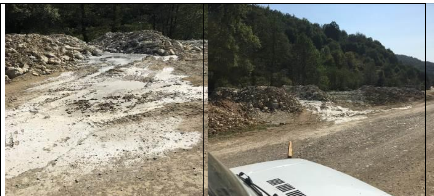
Spilled concrete and mixed (stones, concrete, spoil) stockpiles KM 44+500; 43+980
